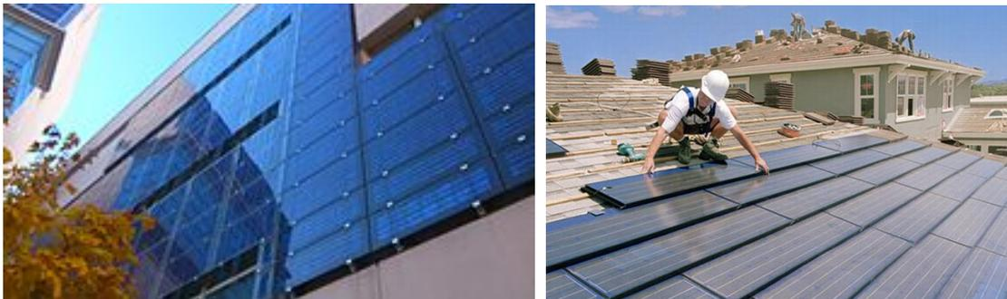
Integrated solar panel in facade (left) [1] and on roof (right) [2]
